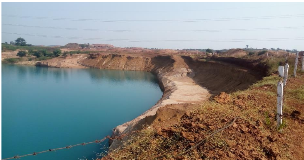
Fig. 3 Mines view photograph
